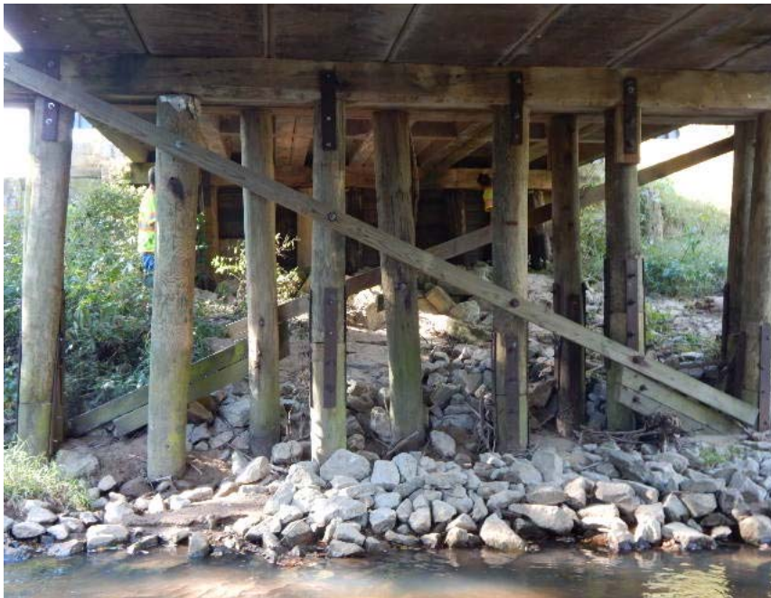
BENT 1 REAR SIDE
