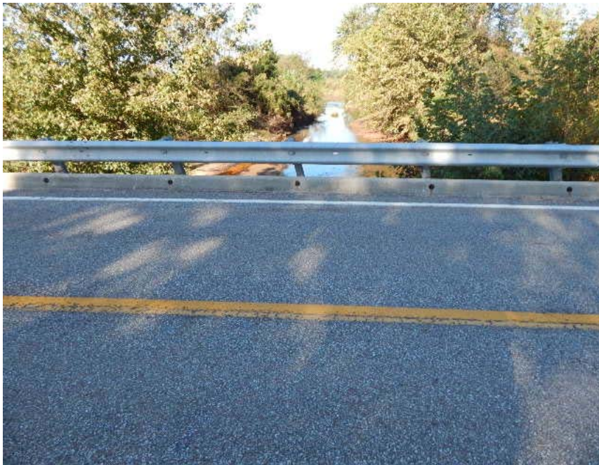
VIEW ACROSS TOP OF DECK
