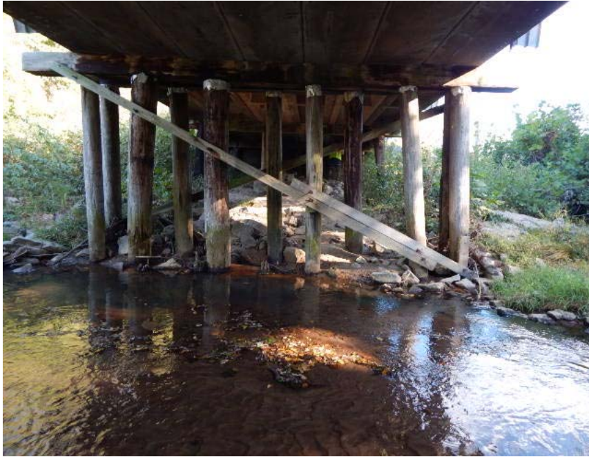
BENT 2 FRONT SIDE
