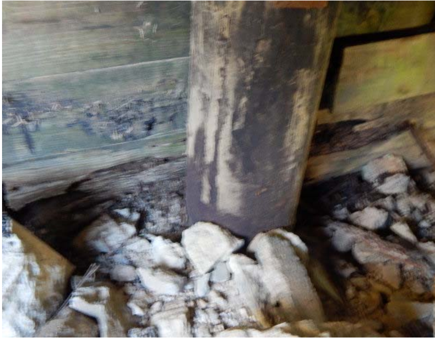
ABUTMENT 2 BREAST WALL
