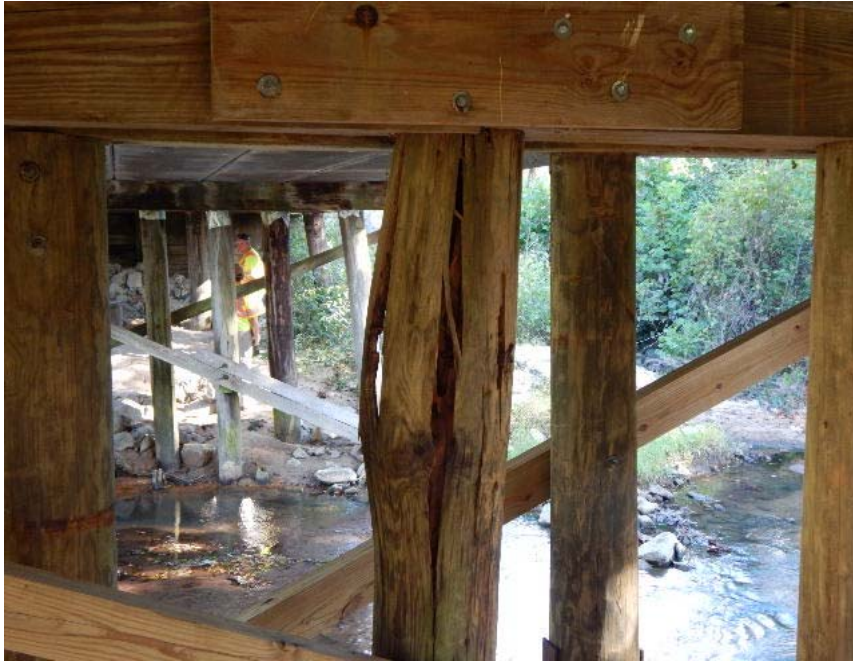
BENT 1 A PILE "C"
