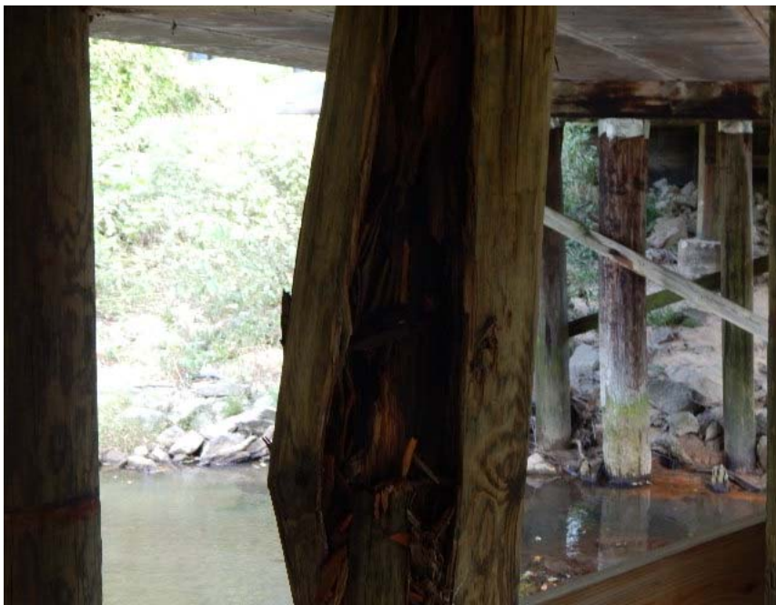
BENT 1 A PILE "C"
