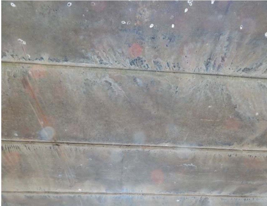
SPAN 2 BOTTOM DECK
