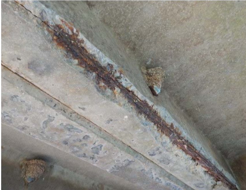
SPAN 1 SLAB "F"
